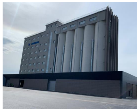
Monfarm - DCF Group – Lucera (Foggia)
