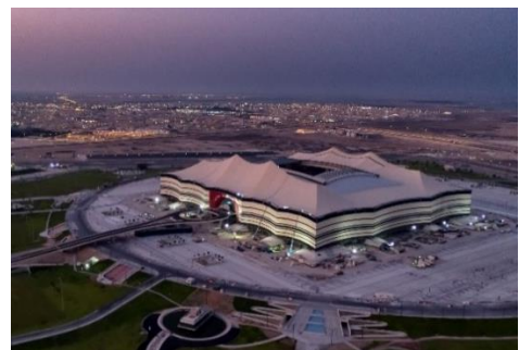
AL BAYT STADIUM in AL KHOR - Doha (Qatar)
